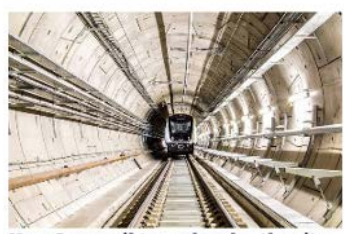
New Crossrail tunnel under the city center. Image Source: Crossrail.
