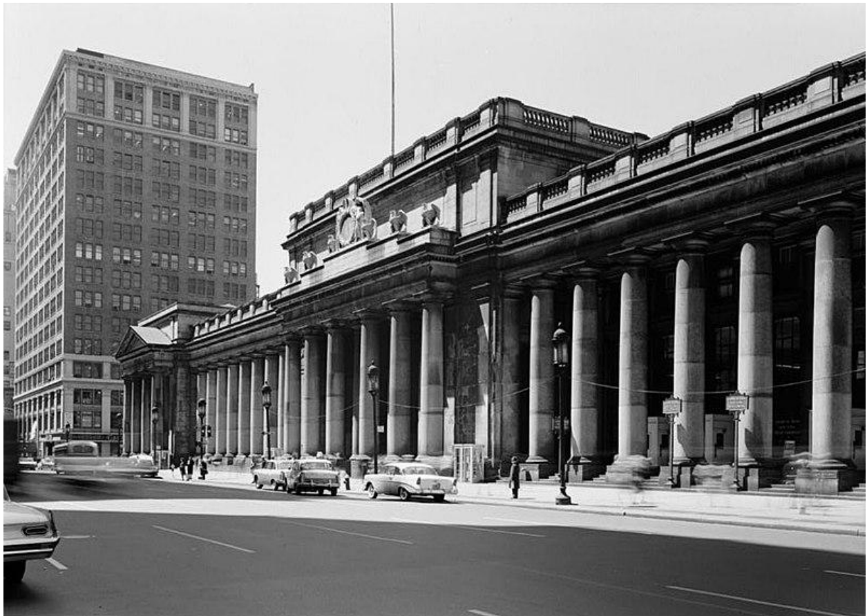
Pennsylvania Station in 1962. Library of Congress via Wikimedia Commons
